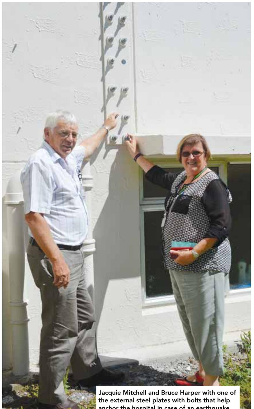
Jacquie Mitchell and Bruce Harper with one of the external steel plates with bolts that help anchor the hospital in case of an earthquake.
